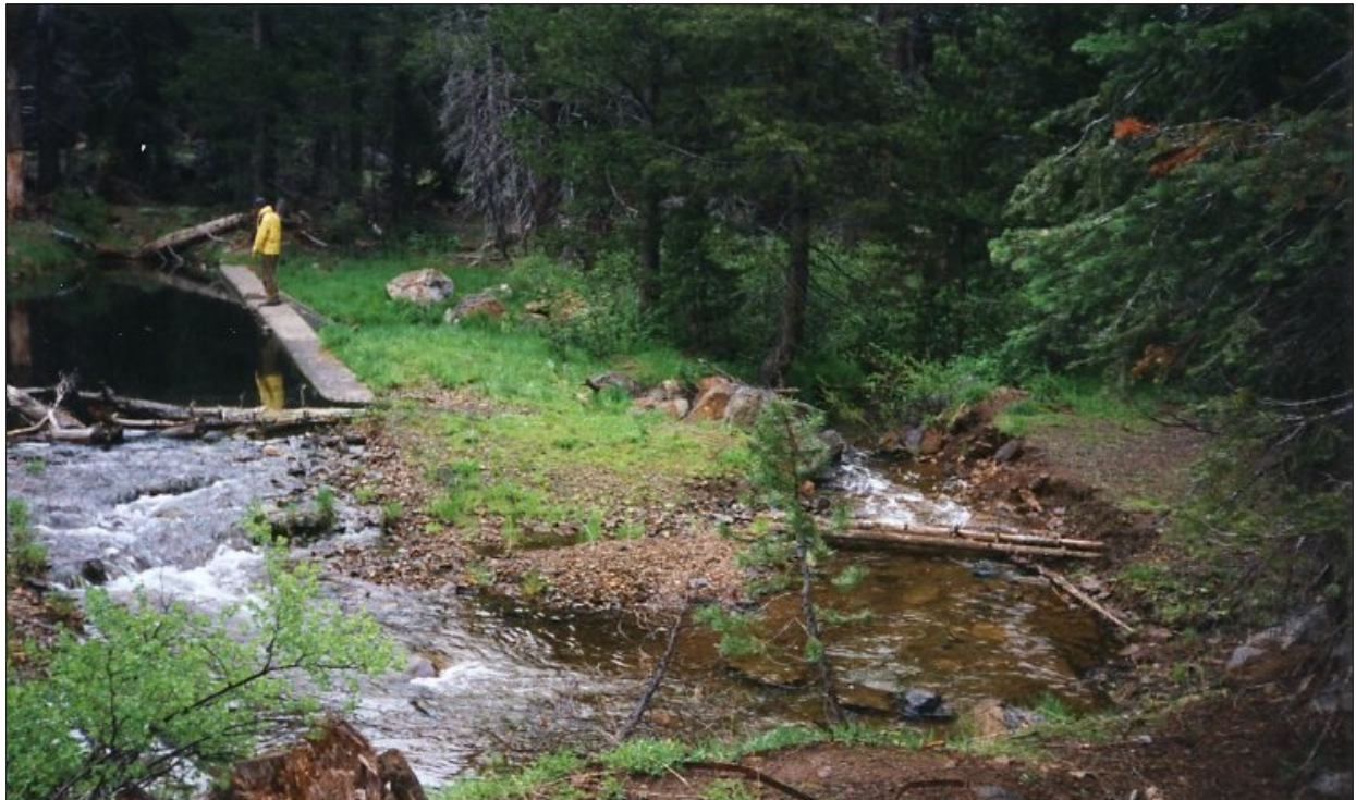
Figure 2. Dam and end-run erosion.
