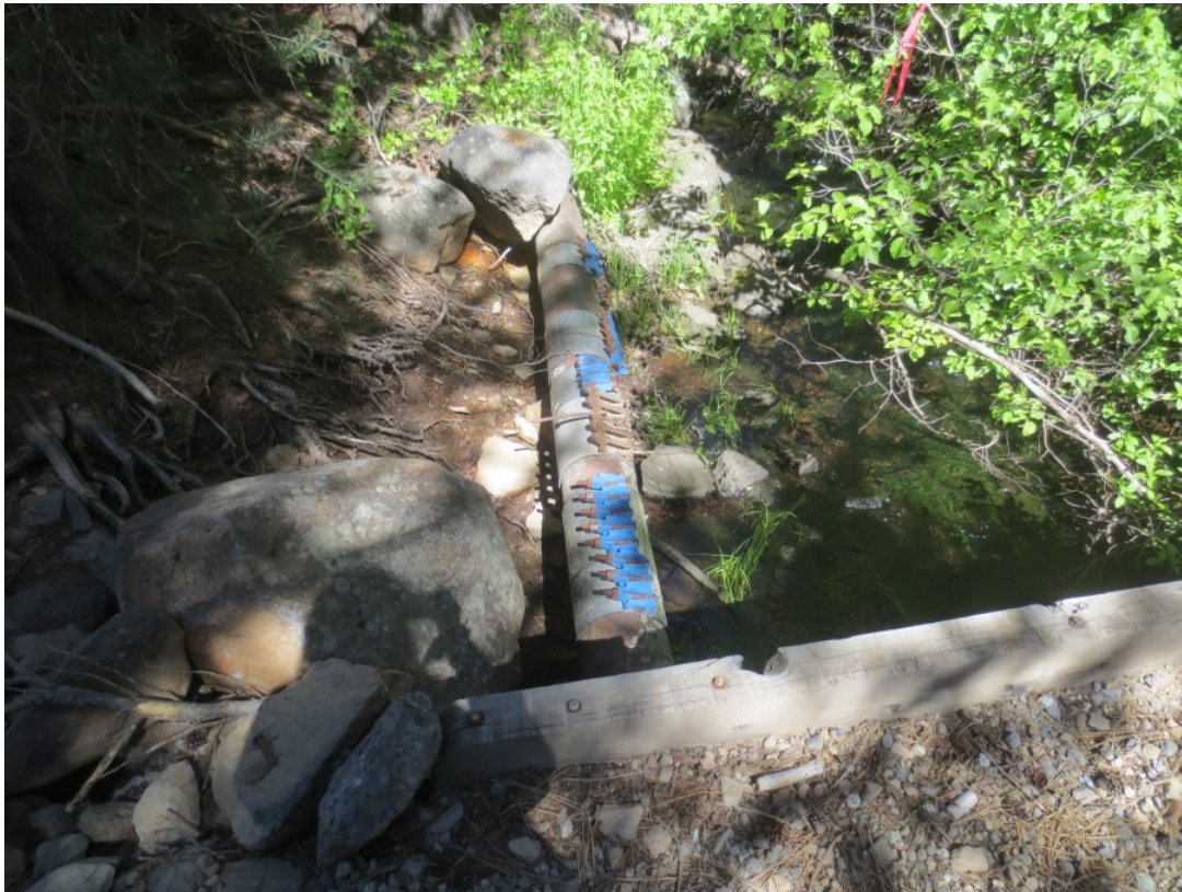
Figure 10. Riveted pipe, with repairs, view south, June 2018.
