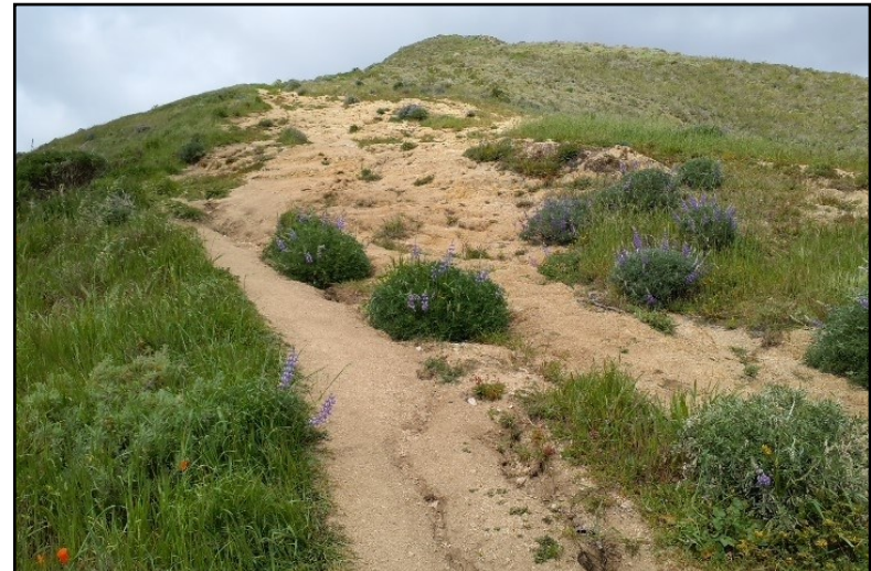
Photo 4. Existing trail ridge, south elevation, showing erosion damage. Photo taken April 12, 2023.
