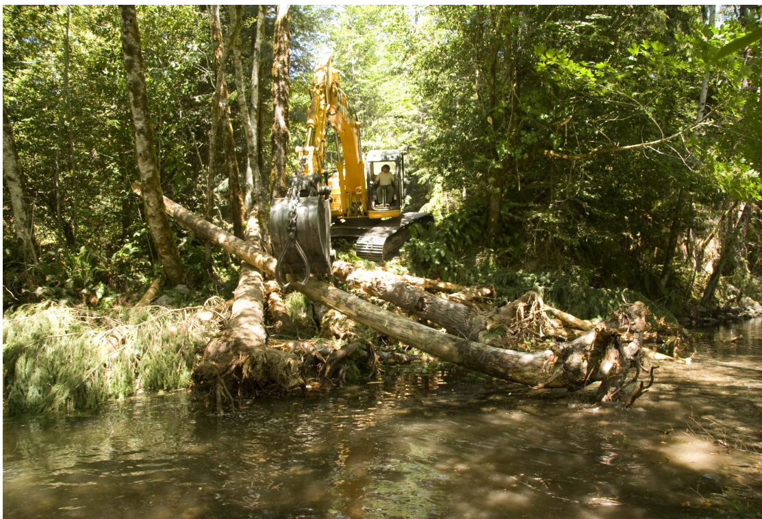
Figure 6. A large wood structure installation in East Fork Mill Creek. September 2008, CDPR.
