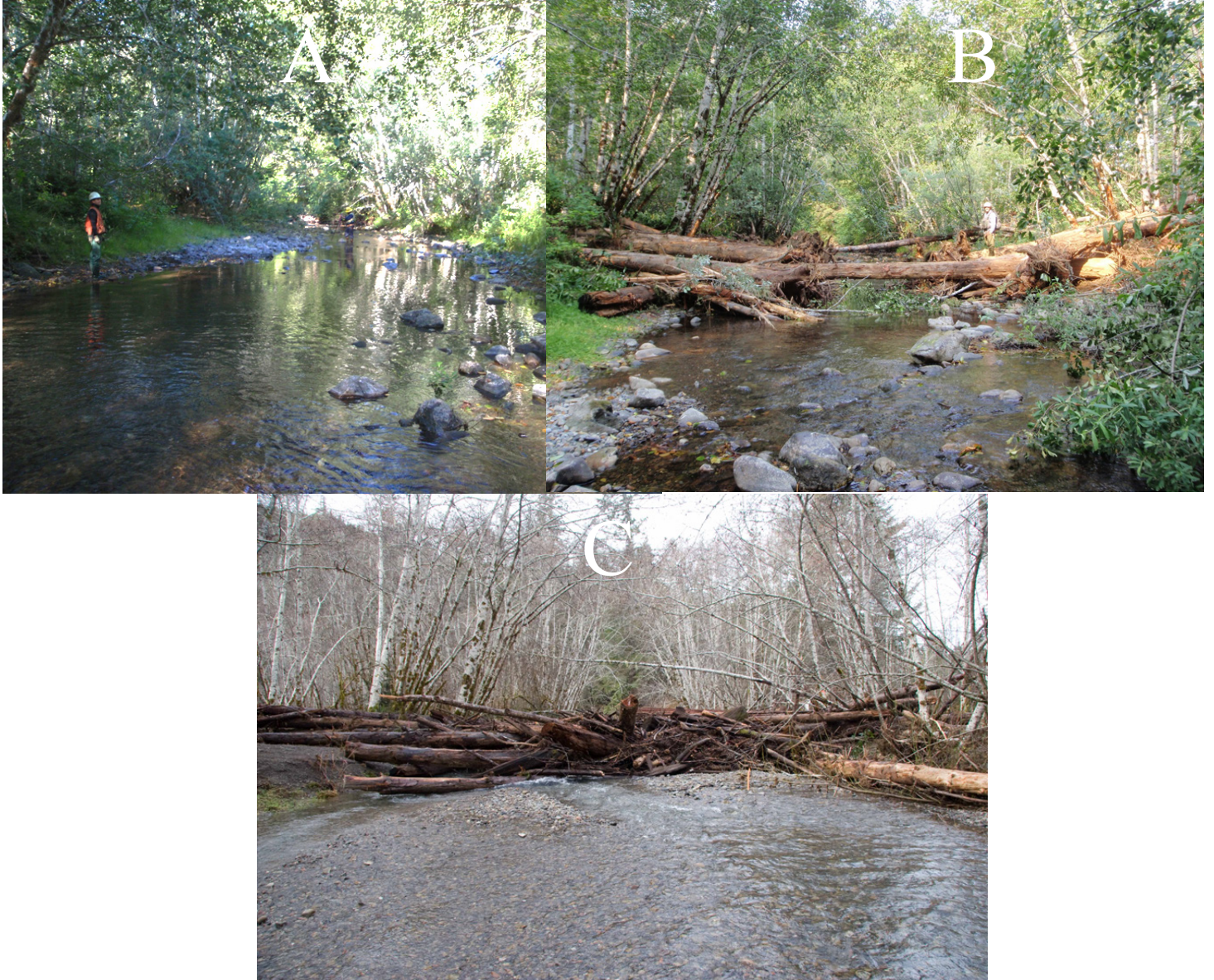
Figure 7. Examples of pre (A) and post (B) large wood installation, and after one winter season post installation (C). Adapted from Benegar 2011.
