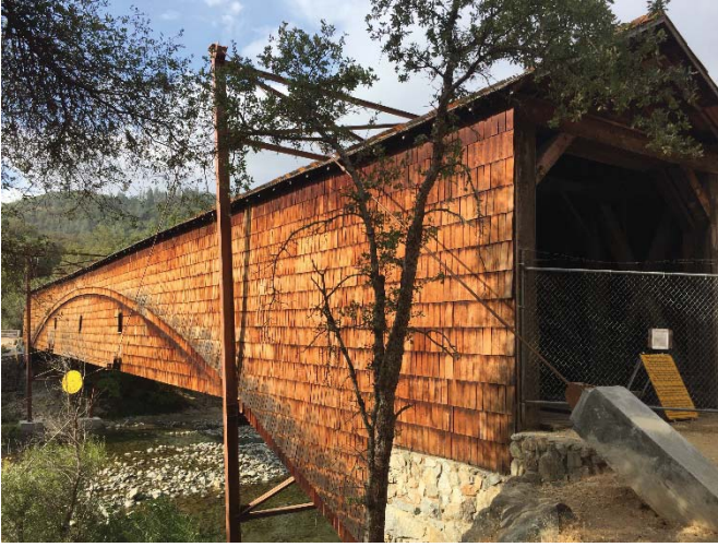
Figure 3: Bridgeport Bridge with Temporary Stabilization Frame
