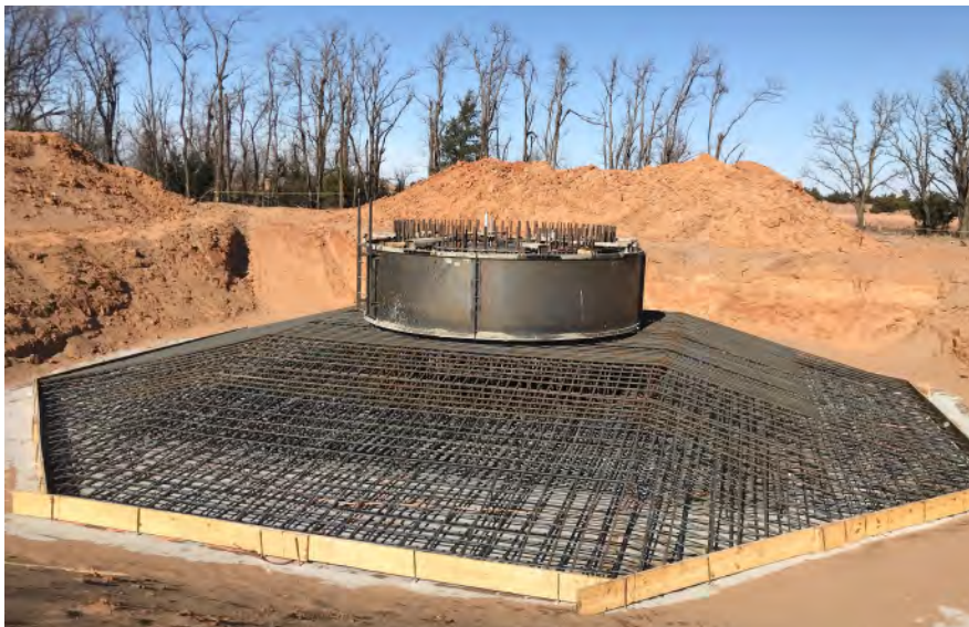
Figure C: Installation of concrete turbine foundation
