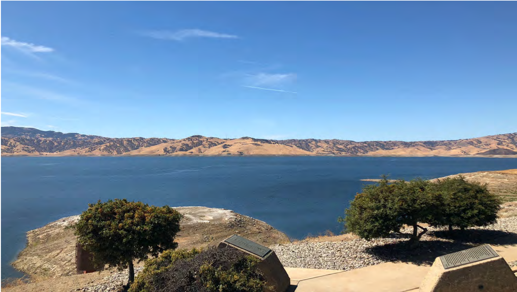
Existing view west from Romero Visitor Center towards project site (located 3.8 miles away - existing wind turbines visible)
