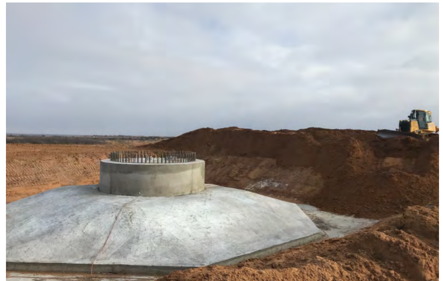
Figure D: Completed turbine foundation
