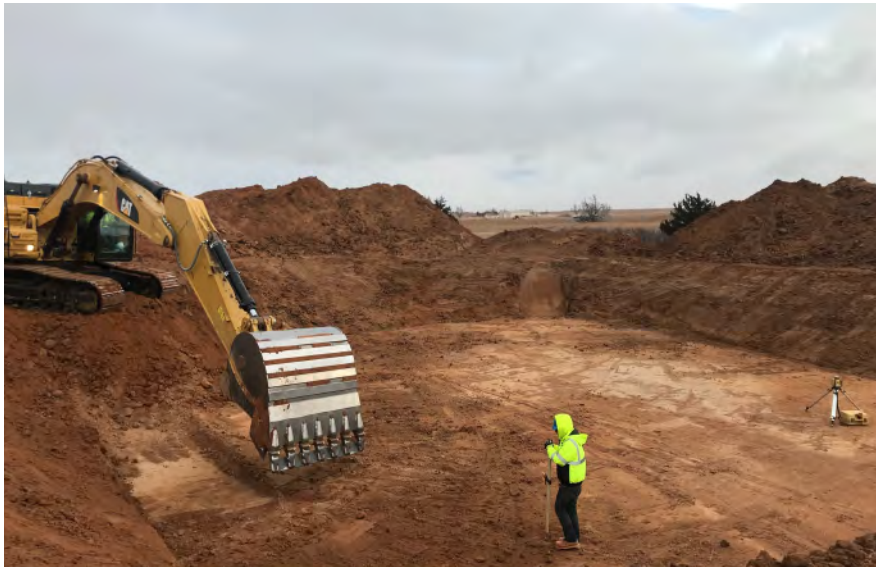
Figure A: Excavation to install turbine foundation
