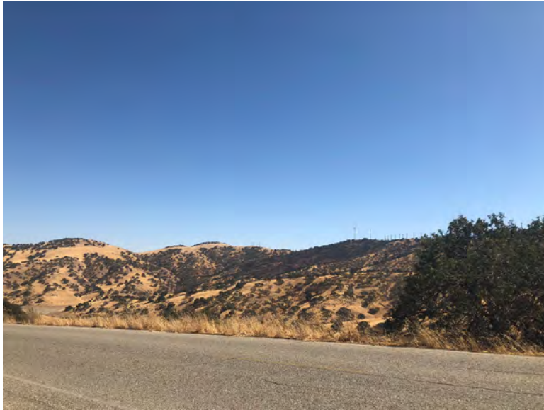
Photograph G: View southeast from Dinosaur Point Road to oak woodland and grassland covered terrain. Wind turbines and a MET tower are visible on the ridgeline.
