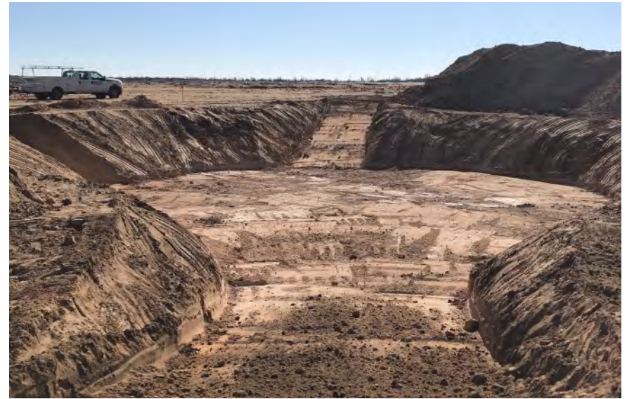
Figure B: Completed turbine foundation site
