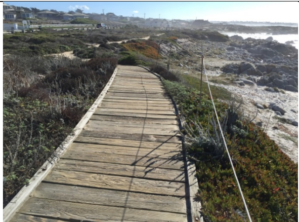
Existing boardwalk to be removed
