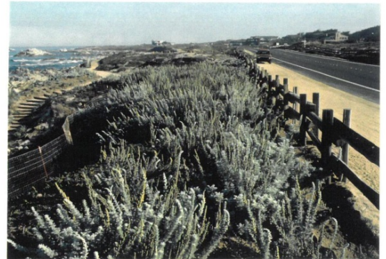
After restoration, the area is both safer and more beautiful.
