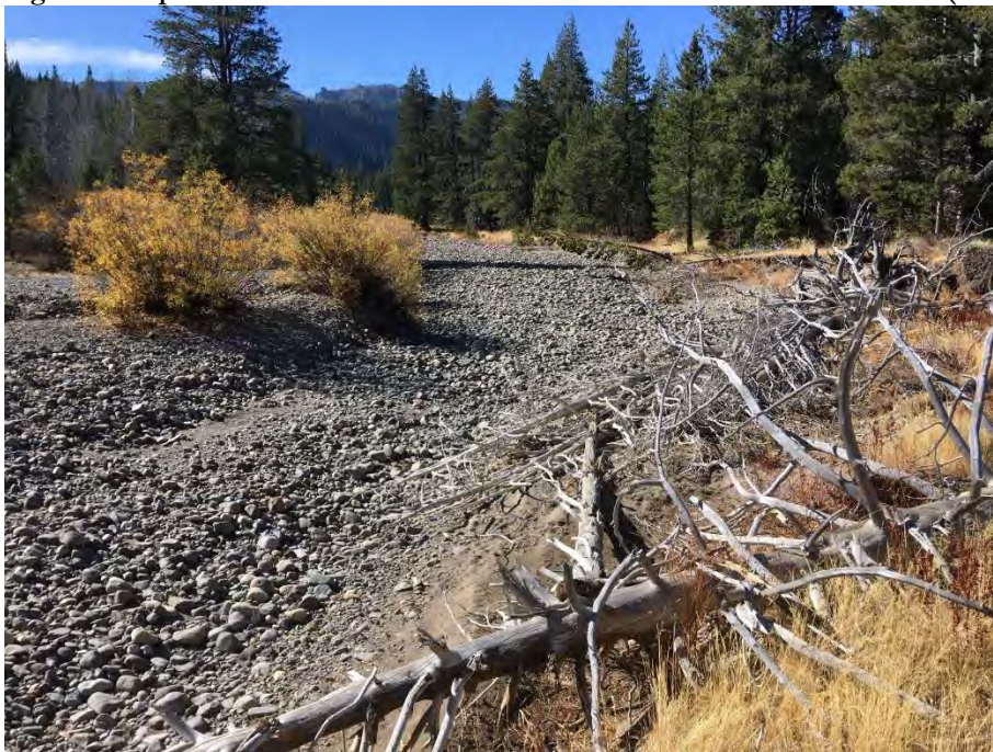
Figure 6. Depositional Zone Downstream from the Railroad Tunnel Culvert (The Chute) (looking upstream)
