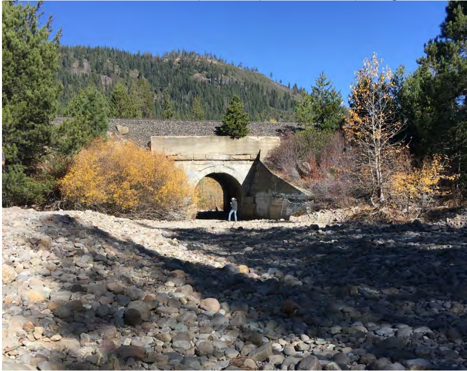
Figure 5. Railroad Tunnel Culvert (The Chute) on Cold Creek (looking downstream)
