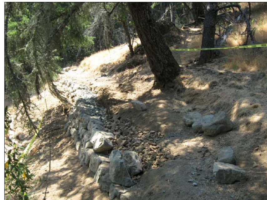
PARTIALLY CONSTRUCTED WALL
