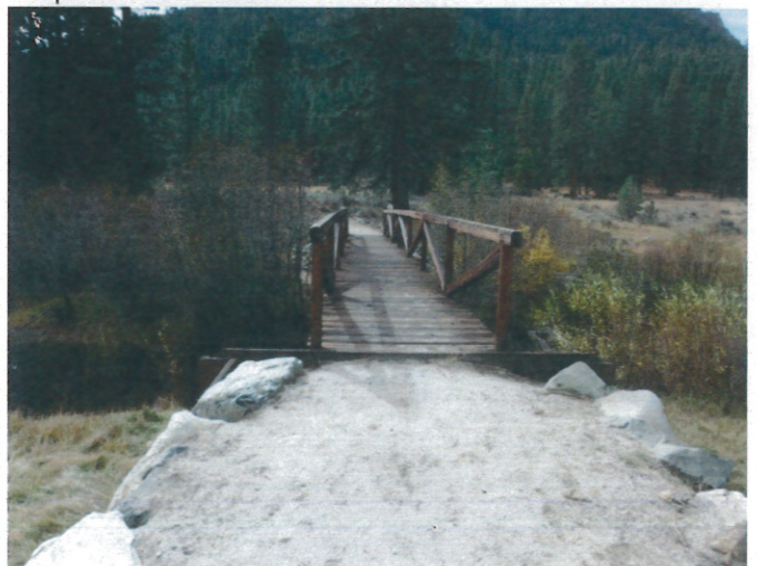
Replace Bridge Deck Planks
