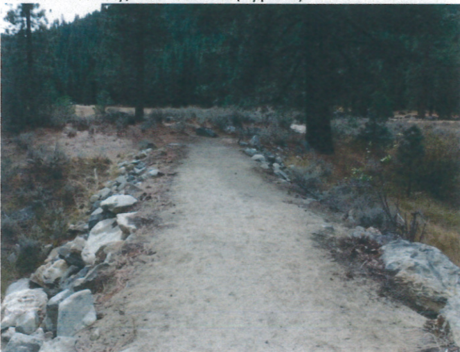
Reconstruct Portions of Existing Retaining Wall
