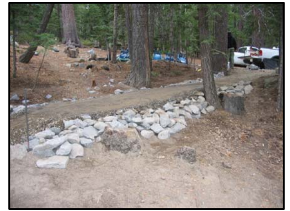
COMPLETED DRAIN LENS
