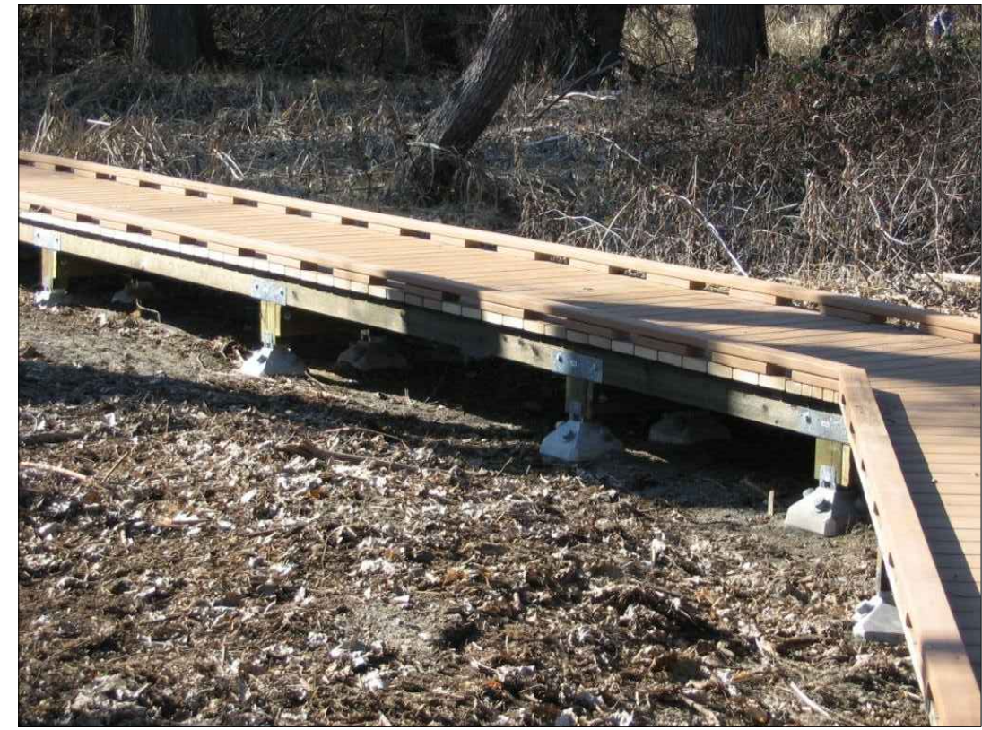
DIAMOND PIER BOARDWALK INSTALLATION
