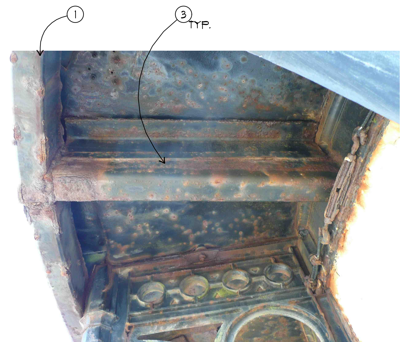
UNDERSIDE OF GALLERY AT EXTERIOR.
