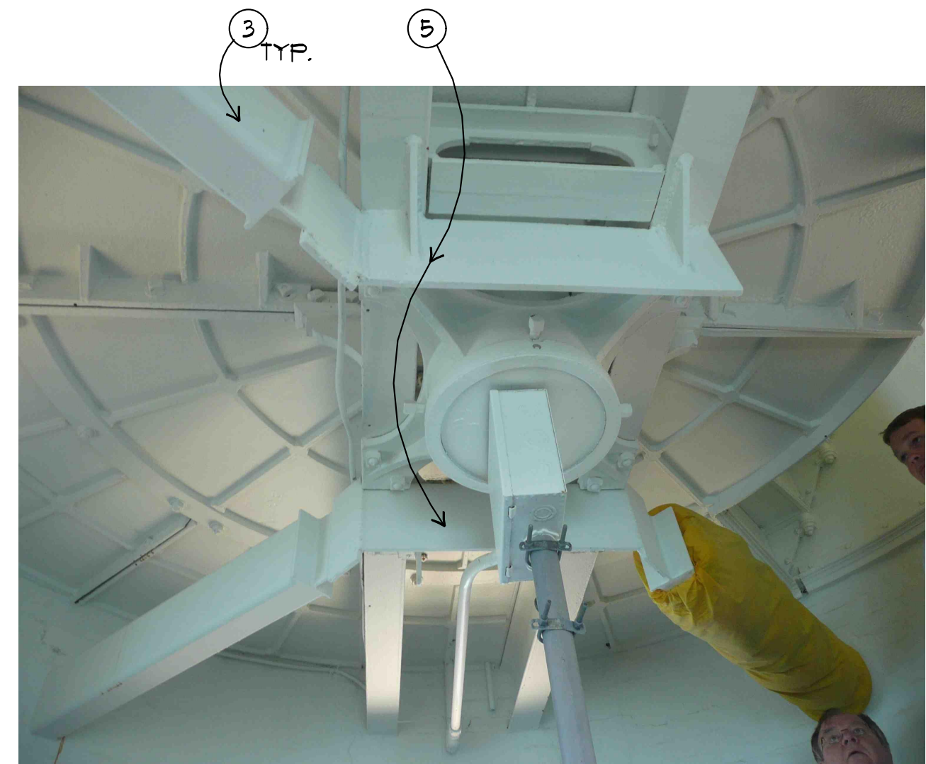
SERVICE ROOM CEILING.
