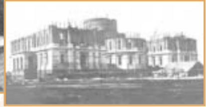
Capitol under construction—1860-74
