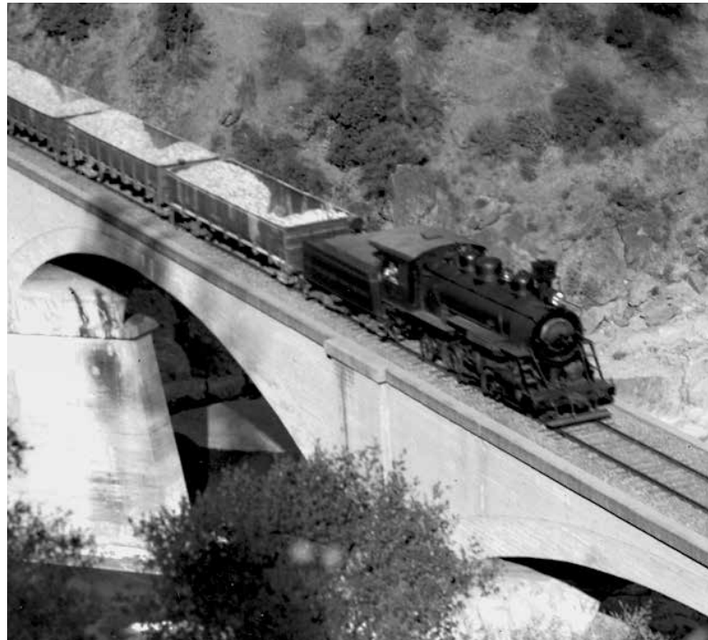
Mountain Quarries Railroad Bridge, circa 1930s
