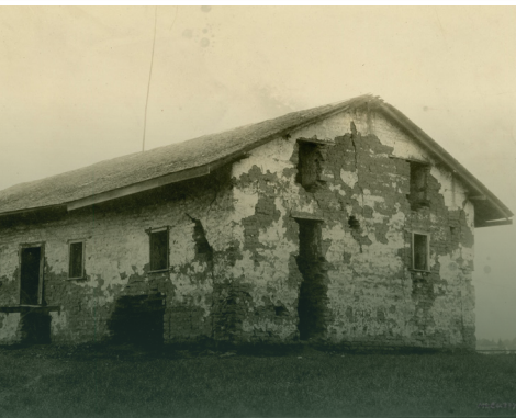
Photograph of the east side of the Central Building at Sutter's Fort prior to restoration, circa 1888.
