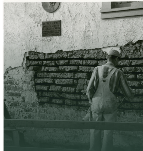
Photograph picturing the restoration of the adobe bricks on the Fort’s Central Building, which took place during the 1950s and 1960s.
