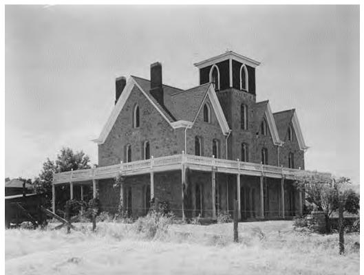
Figure 2: View of the east (right) and south (left) walls of the house, c. 1925. This photograph illustrates the shortened chimneys and the last of three tower and piazza designs. (Source: Historic American Buildings Survey, National Park Service)
