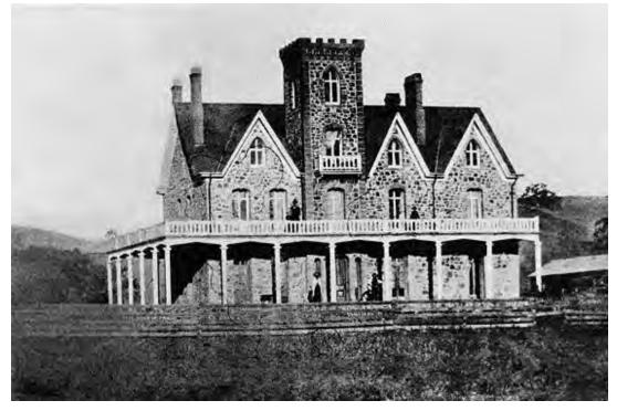
Figure 1: View of the primary or east wall of the house, c. 1856-1868. This image shows the original piazza, brick chimneys, stone tower and balcony at the first level of the tower (Source: Historic American Buildings Survey, National Park Service)
