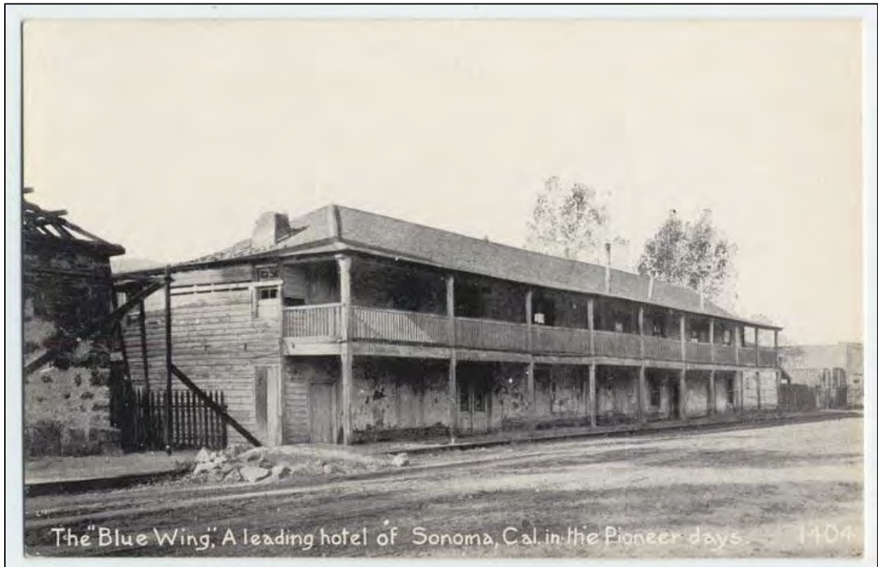
Image 27: Blue Wing Inn, early 1900s. (Courtesy of Bancroft Library, U.C. Berkeley).
