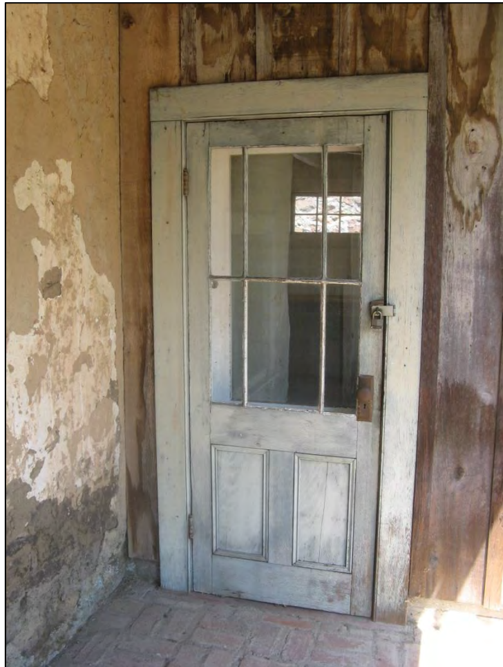
Image 47: Rear kitchen door at the Blue Wing Inn.
