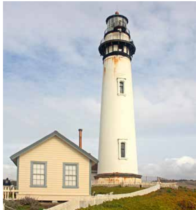
View of Lighthouse and Carpenters Shop from overlook behind the Fog Signal Building.
