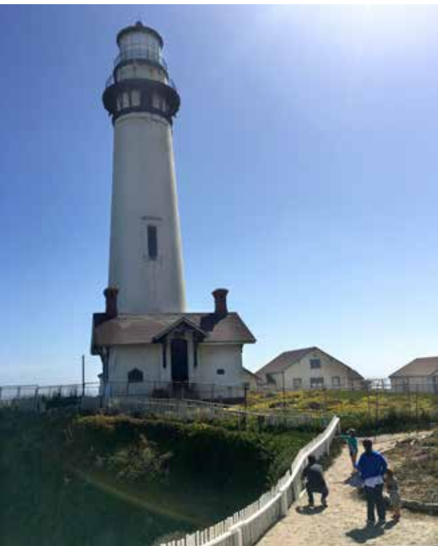
Lighthouse and attached oil house.
