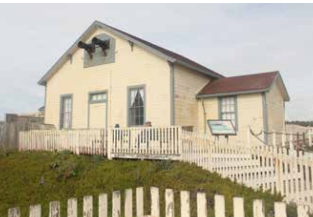
Fog Signal Building (west facade) and viewing deck.
