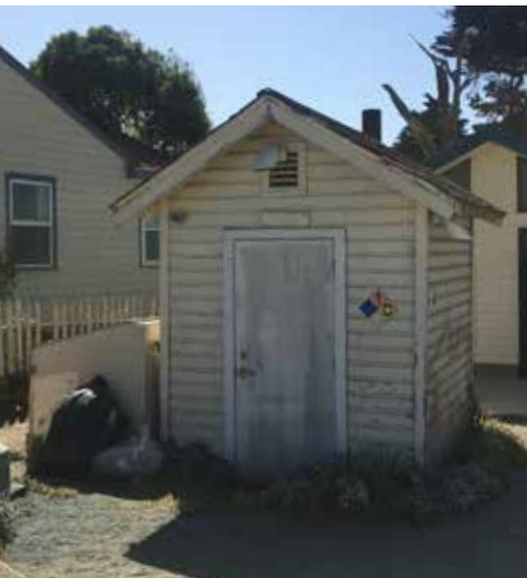
Water Sand Filter Building.
