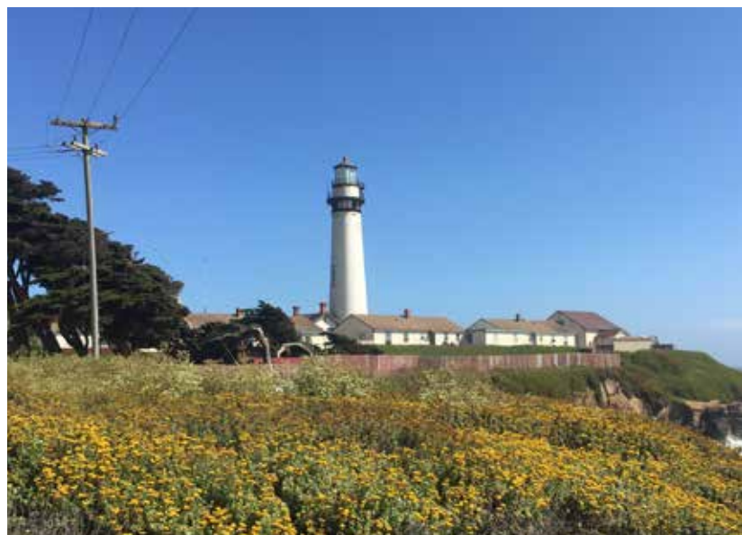
Utility poles along Pigeon Point Road detract from views of the Lighthouse.
