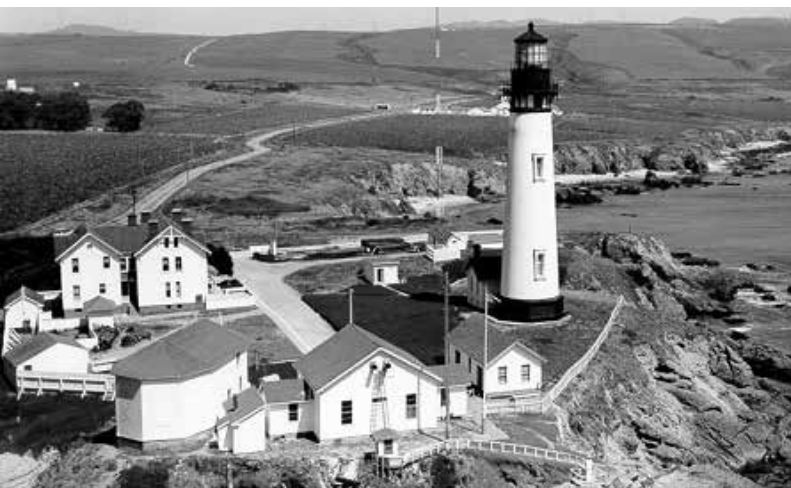
Historic Photo of Pigeon Point Light Station (source: United States Coast Guard)
