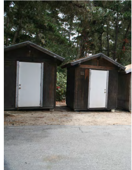
Storage facilities at Rat Hill maintenance and operations area in the Reserve
