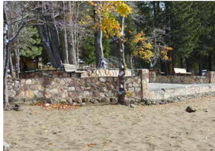
Aging Walls and Stairs
