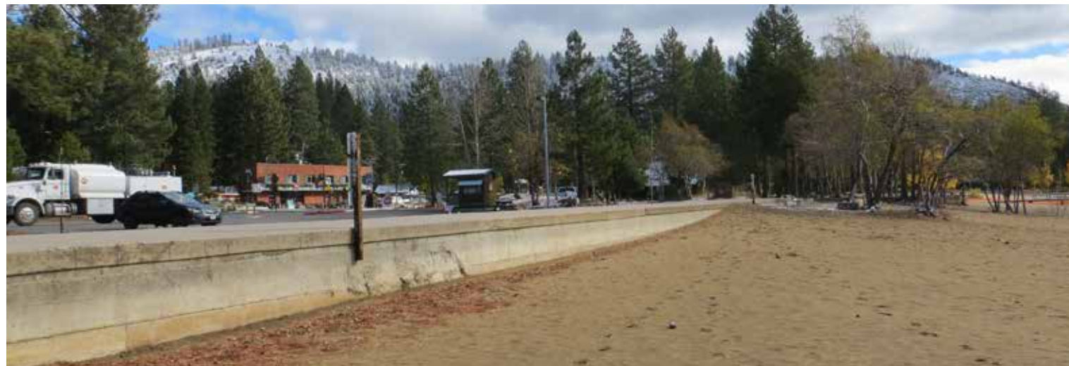
Retaining Wall along Parking Lot and Walkway
