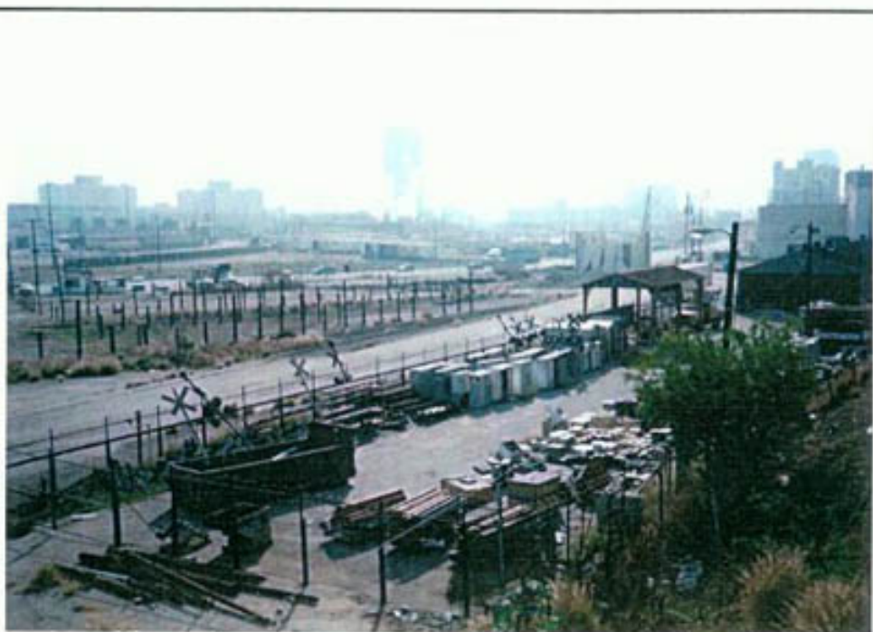
View of subject looking down from Broadway at north end.
