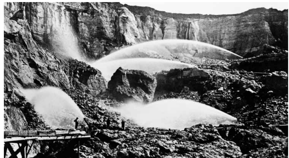
High-pressure monitors wash gold from rock at the pit.
