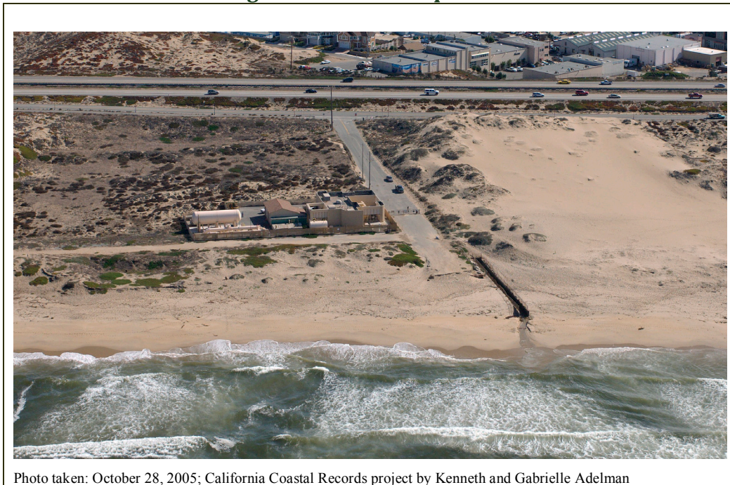
Figure 25. Seaside Pump Station
