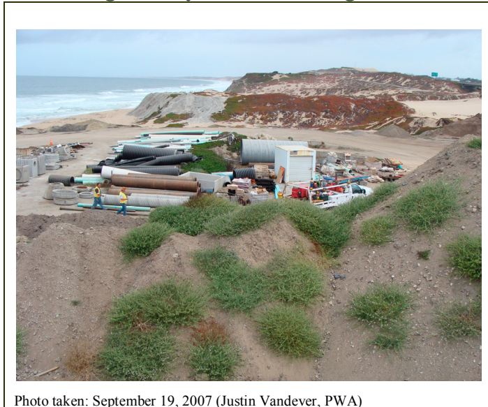
Figure 24. Storage Facility at the end of Tioga Avenue, Sand City
