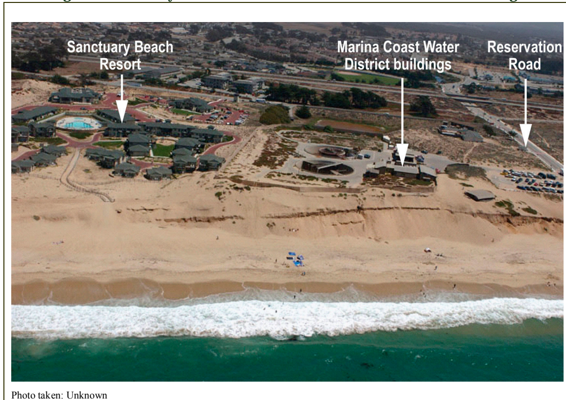
Figure 23. Sanctuary Beach Resort and Marina Coast Water District Buildings
