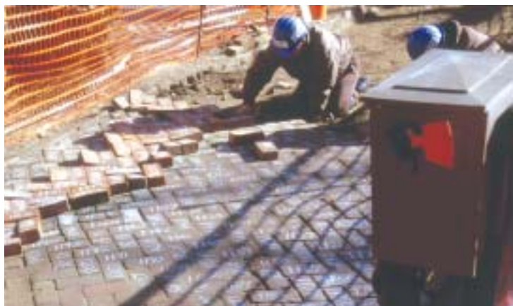
California Conservation Corpsmembers laying historic brick at Stanford Mansion State Historic Park
